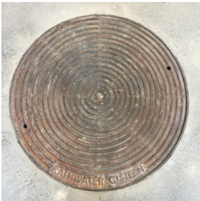
Rainwater collected in cisterns will be used to flush toilets (natural color variation may occur!).
